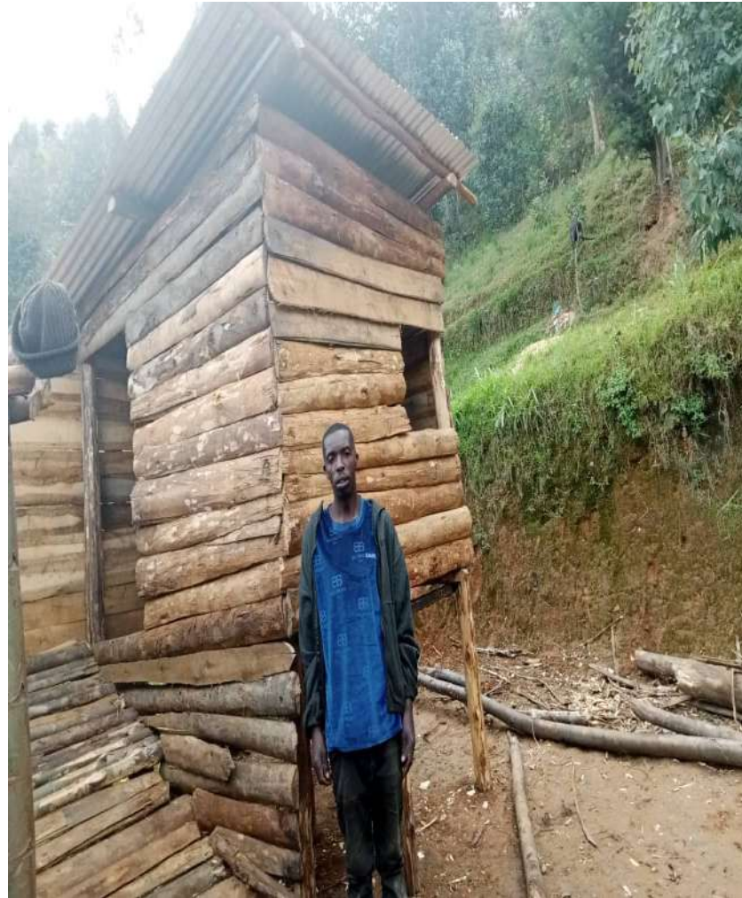
Raised shelters construction
